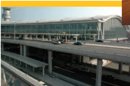
Terminal 1, Pearson International Airport
